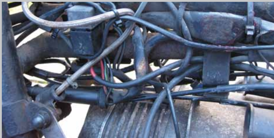
Although the hacked about wiring in the headlamp bowl benefited from some attention, the electrical fault was actually hiding here, under the starter relay
